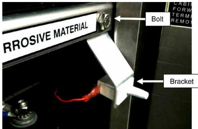
47. Make sure the switch engages when the battery cabinet door is closed. Close the battery cabinet.
