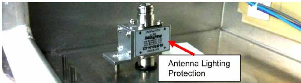
**NOTE:** The rubber ring gasket goes on the inside of the cabinet. The marked text "Antenna" points down and "Equipment" points up.
