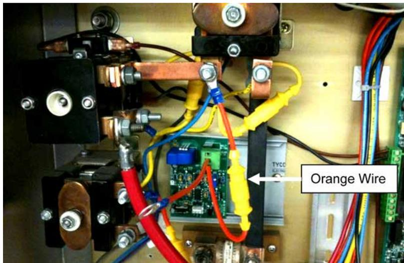
15. Remove the nut 7/16 inch. Remove and discard the orange wire.
