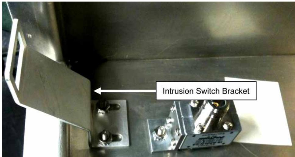
37. Install the intrusion switch (item 10) using a 3/8-inch socket.
