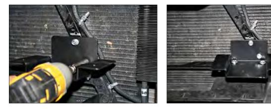
5. Align the AS124 speaker on the mounting bracket. Secure it from the top with two 1/4"-20 bolts and 1/4" flat washers and from the bottom with two 1/4" flat washers and lock nuts from the bottom.
