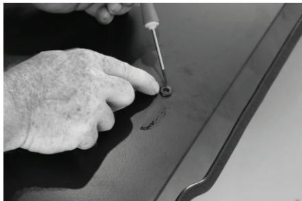
Figure 6 Install grommet
