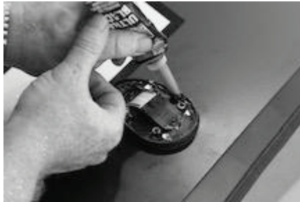
Figure 18 Fill grommet hole and base with RTV or silicone
