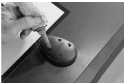
Figure 20 Fill holes with RTV or silicone
