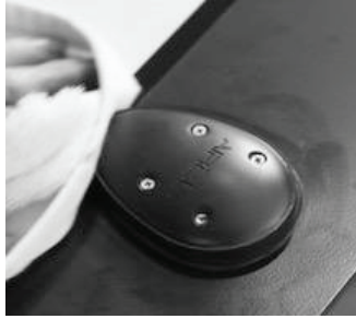
Figure 24 Wipe off excess RTV or silicone
