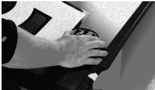
Figure 3 Position housing pod and mark hole
