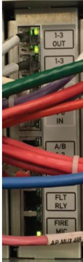
14. Write down or photograph the labels and connector positions of all the cables exposed by the removed front cover.
