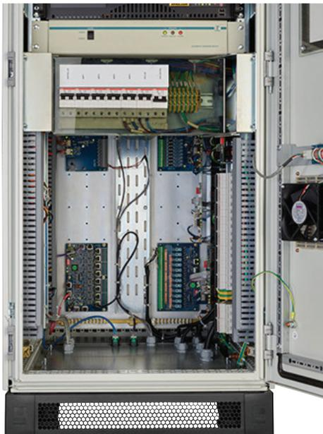
The MDF contains three areas for mounting terminating equipment: left panel, right panel, and back panel. The left panel is used to mount amplifier audio distribution terminal cards for loudspeaker terminations. The right panel is used for power terminations and mounting the Beacon Monitored Output card. The back panel is used to mount any of the system I/O cards.
