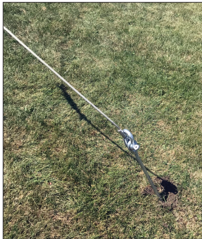
Figure 64 Cable attached to the ground anchor
