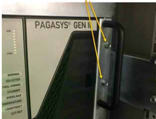
Figure 65 Removing the chassis mounting screws
