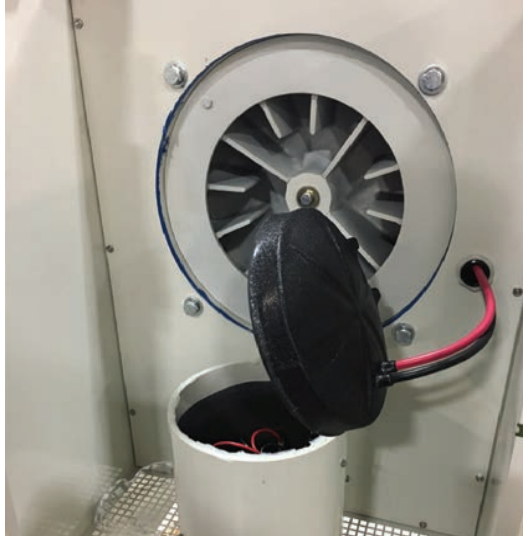
Figure 19 Installing new black cover
